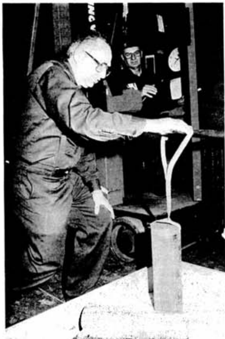
Gil Roy, storeman in Divisional Shops, left, doesn't have to manually lift scoop bucket pins anymore thanks to a new ergonomically-designed strap that allows the heavy pins to be lifted by forklift. Moving the pins, weighing as much as 120 pounds each, used to contribute to painful back strains. Forklift operator and storeman Reg Selle added, "You feel more secure lifting the pins because it's a lot safer. I know the strap won't fall because it's designed for the job."
