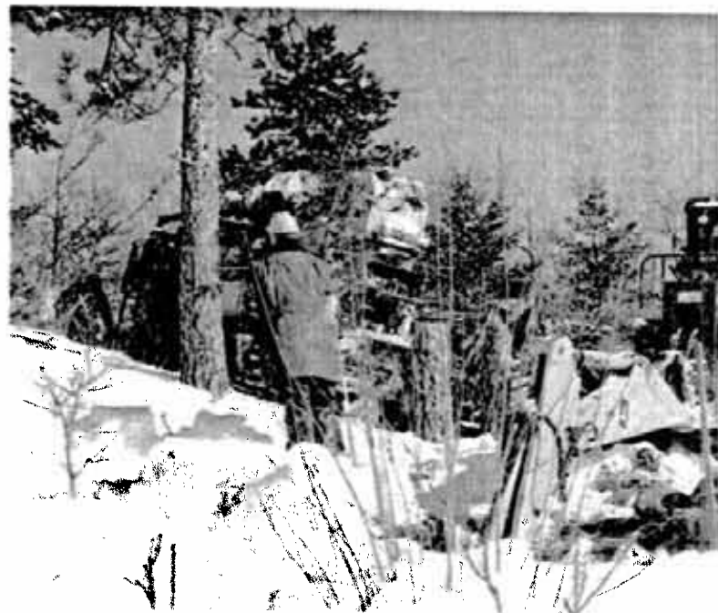
Lead hand Steve Fournier (back to camera) watches the go-to swing a new pole towards him for placement in the hole
