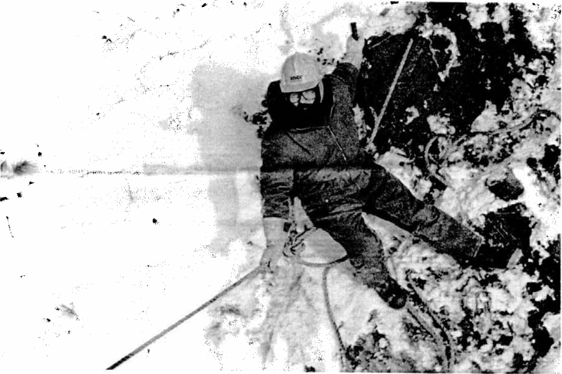
Line foreman Claude Mailloux keeps tension on the guy rope used to support the pole while a co-worker works above.
