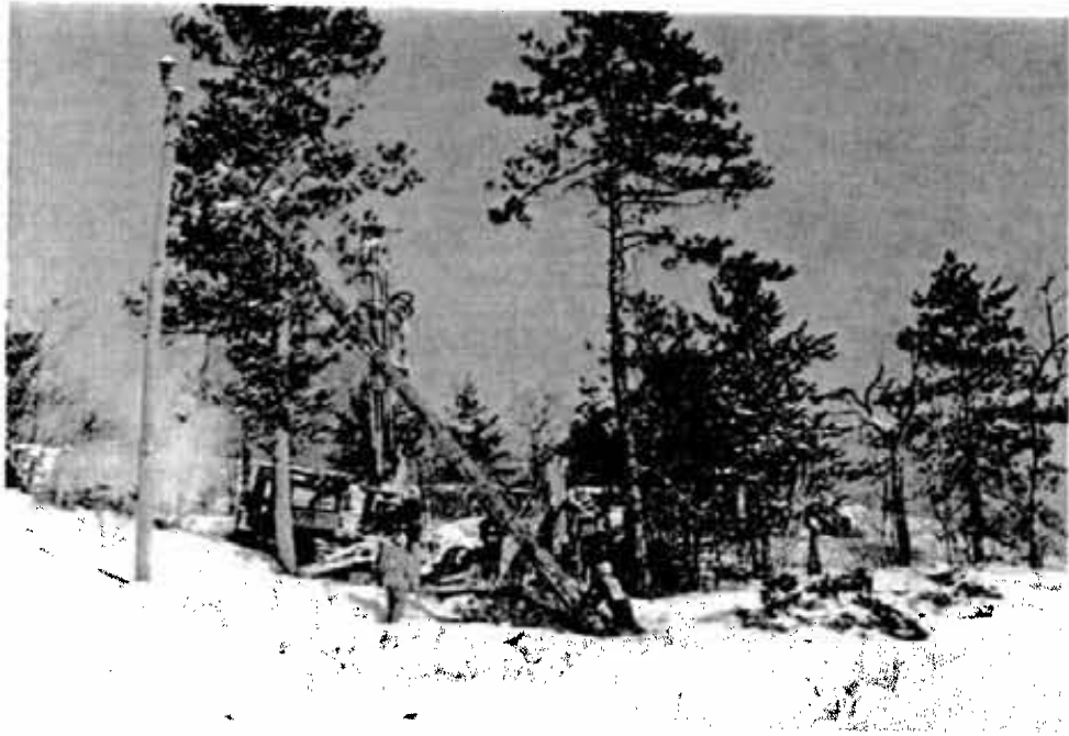
Crew members work to erect a new pole on the hillside.
