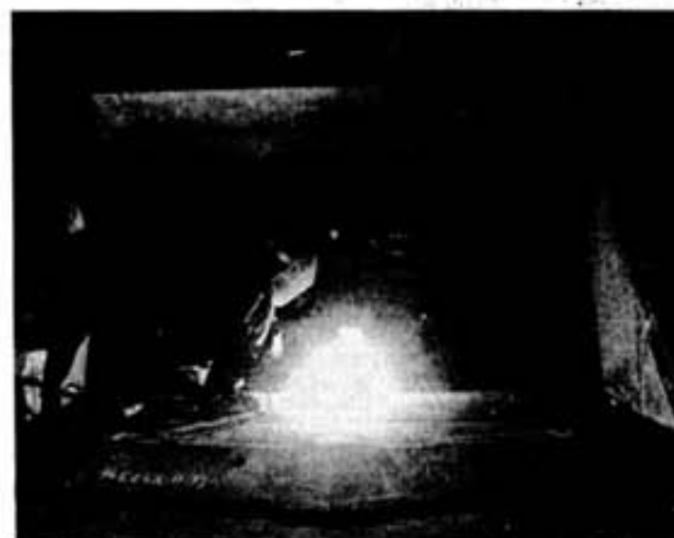
Welder Jarl Paavola works on a repair inside a bucket at the Heavy Equipment Repair Shop.
