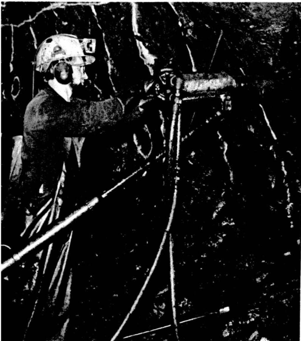
Roger is pictured doing what he does best at Copper Cliff south mine, operating a jack leg in a stope.
