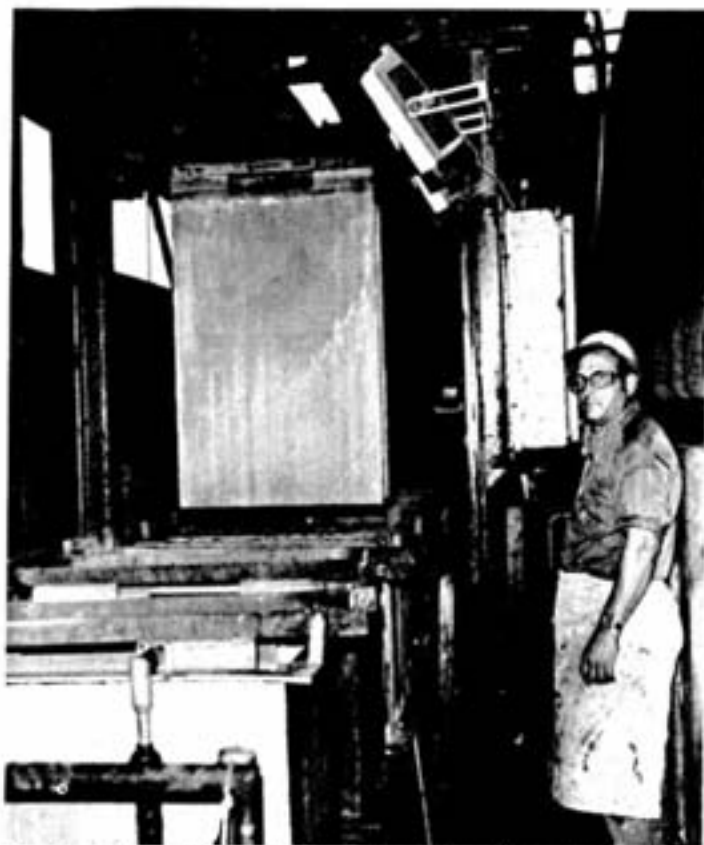
The ink is stripped off the sheets, or "mandrels" then recoated after approximately every six cycles in the plating tanks. Looking on is Ettore Guglielmi.
