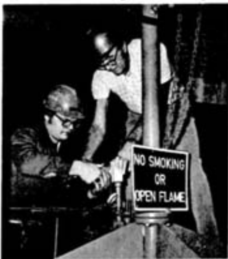
The installation of the submerged combustion evaporator in the electronic refinery at Port Colborne has been completed. The new equipment introduces a natural gas flame directly into the electrolyte, bringing its temperature up without the introduction of steam which added water. In addition, this equipment can act as an evaporator to assist in controlling electrolyte volume. Above, from left, Neil DeKoning of the engineering department, and Roop Bahn check final installation details. Below, Bill Lewis left, and Len Richards , of the instrumentation department, are working on the flame igniter.
