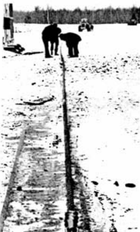
Here the rope is being pulled off the hoist drum by front-end loader.
