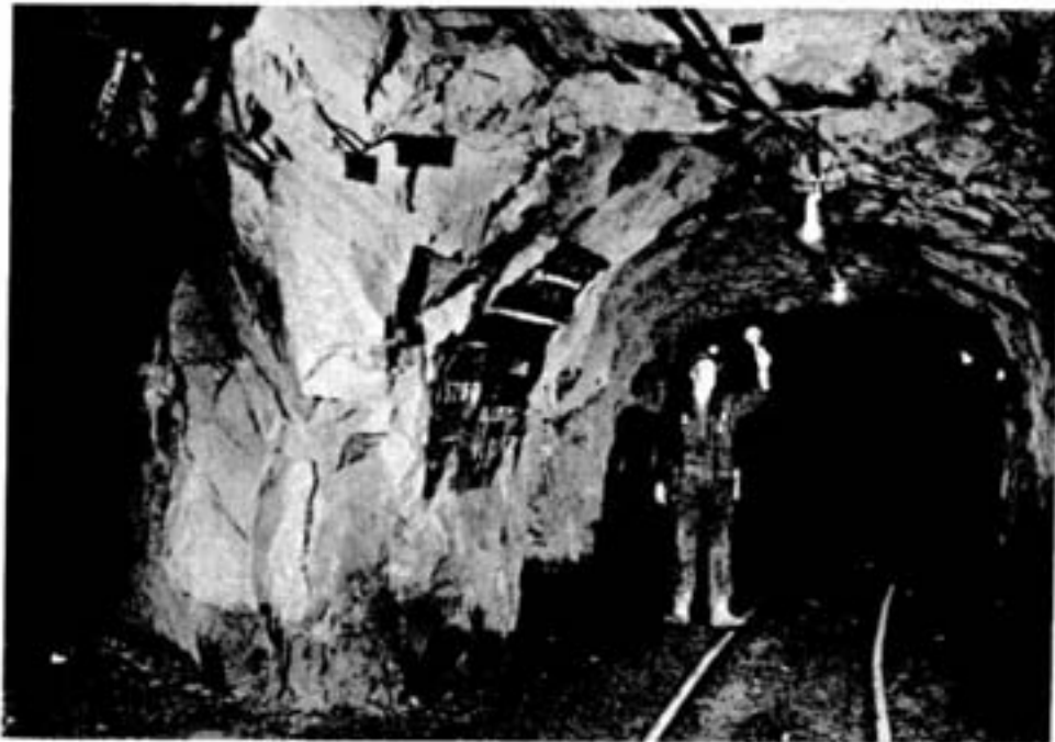
Frank Reynolds, ventilation supervisor at Stobie, is using an anemometer to measure the split of air volume through 7 shaft crosscut at the main haulage drift on 1800 level. Regular checks are made on air flow in all areas.
