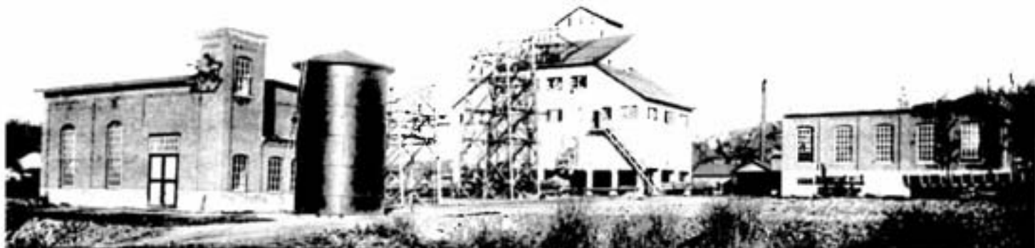
The surface facilities from Crean Hill's first production era are shown above, with the headframe and rockhouse at centre, the old hoist house at left and between them the idler towers, over which the hoist cable ran.
