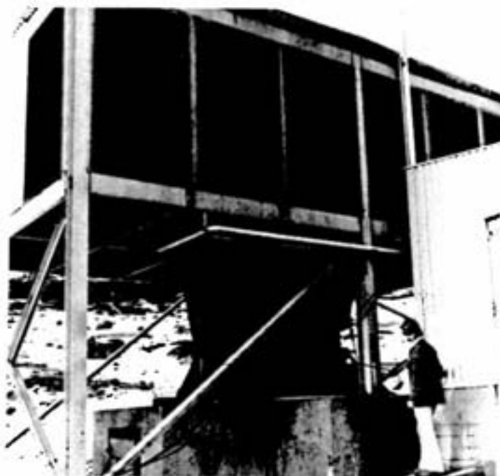
This is one of Frood's fresh air fans. Using a manometer, Keith Rogerson is checking the static pressure at the fan intake to determine if there is any restriction to the flow of heated air down the shaft.
