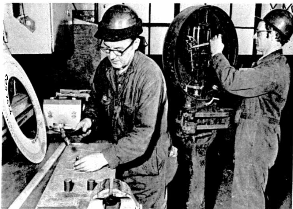
Back in the shop, Elvin fabricates a jig to make replacement links for the 100-ton railway scale, while in the background Stew overhauls one of the plant's older dial scales.
