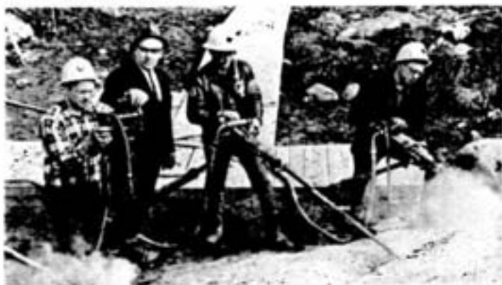
Under the watchful eye of their instructor, Joseph Bardswich, P.Eng., three mining technician students, Pete Morrison, Bob Sipprell, and Will Grant carried out a drilling, loading, and blasting operation on a rocky outcrop behind the college.
