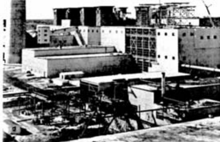
Extension of the smelter, shown almost completely sheeted in, is being carried out in two stages. Two converters, a 32-kva electric furnace, a fluid bed roaster, two filters and a thickener are being added in 1968. In 1969 another converter, another 32-kva furnace, a filter and two thickeners will be installed.
