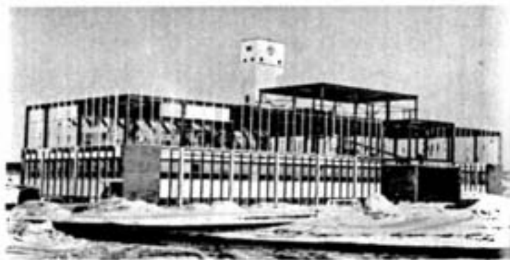
The expansion program has stepped up the already pressing need for additional office accommodation at the Thompson plant, and the administration building is getting an extension to the back wing and a second storey all around. Building services will be installed in the penthouse. The top of the T-1 shaft headframe appears in the background.
