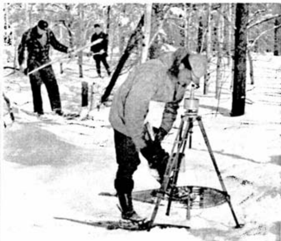
Geologist Percy Sheppard takes a reading from the magnetometer to record Mother Earth's "pulse" at this particular spot in an area which is being explored for nickel-bearing ore. The stake over which the tripod is centred indicates a 200-ft. snark on the base line previously laid out by the survey party. In the background Walter Jarvis and Percy Castonguay clear out a cross line at right angles to the base line.
