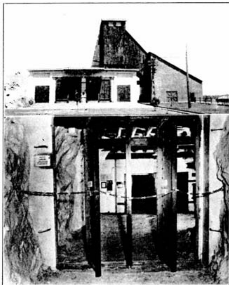
Major features of Frood's ventilation setup, described in the accompanying article, are pictured here. Top photo shows the headframe, hoisthouse, and fanhouse at No. 1 shaft. In the fanhouse (foreground) are the two huge fans driven by 450-h.p. motors, which send 468,000 cu. ft. of air per minute to the underground workings. Pictured below is a shaft station at No. 1 shaft (this one is on the 2800 level) which receives the fresh air from the shaft for the level. In the immediate foreground are the butterfly doors which can be adjusted to regulate the amount of air to the level, and at the shaft opening inside the station can be seen the louvre doors, also adjustable and used to regulate the supply of air.
